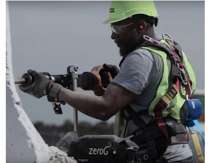
Exoskeleton for Construction, Ekso Bionics
